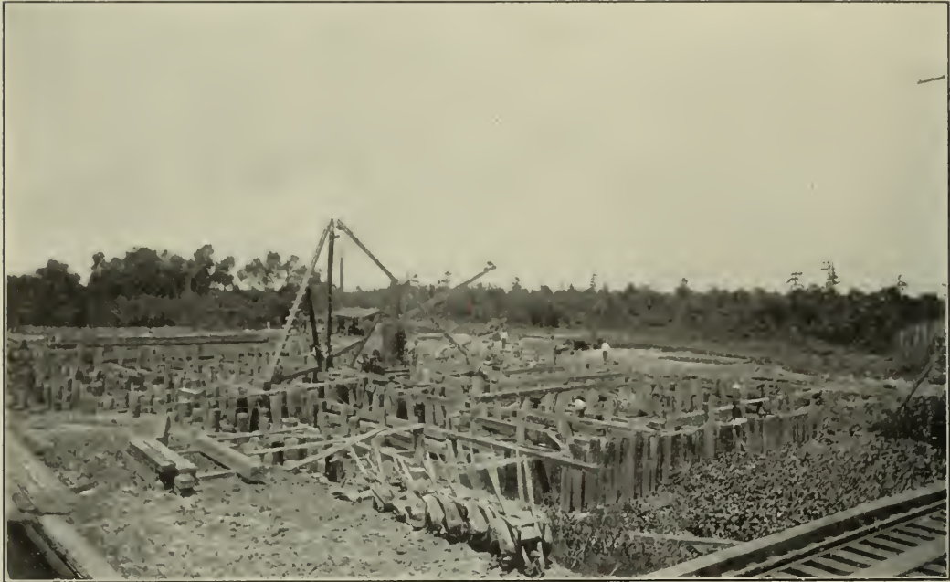
THE PILE-DRIVEN FOUNDATIONS FOR PUMPING STATION NO. 7 APPROACHING COMPLETION.
